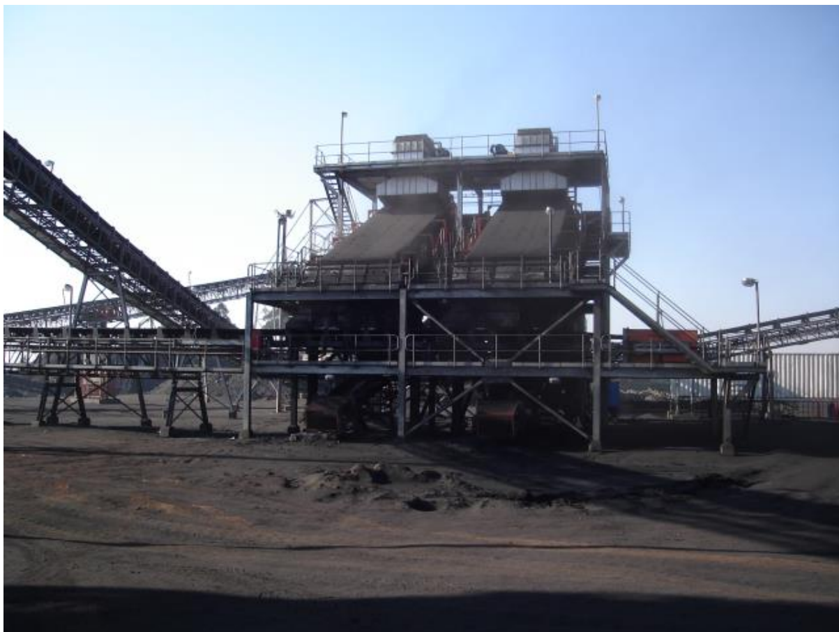
Figure 10: Liwell screens for dry screening of coal
